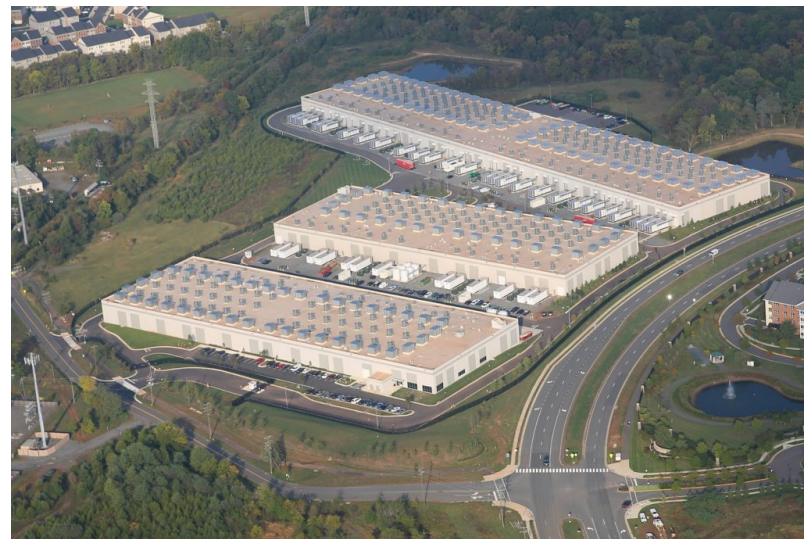
Northern VA datacenter
